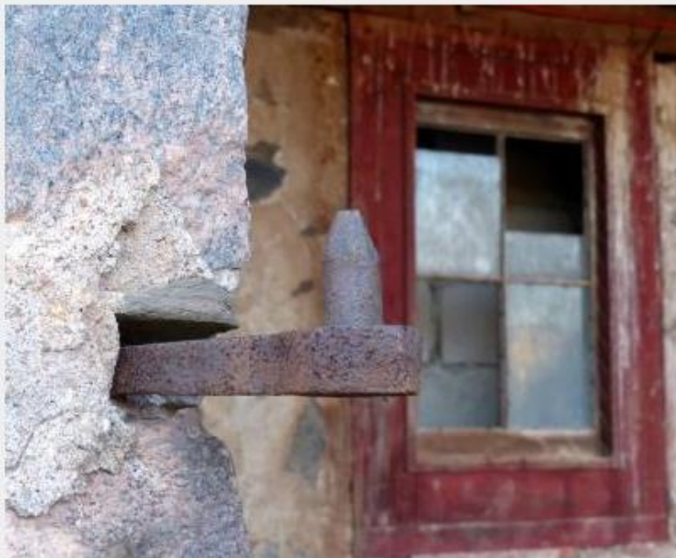
Pintle - embedded gate hinges in a stone wall
